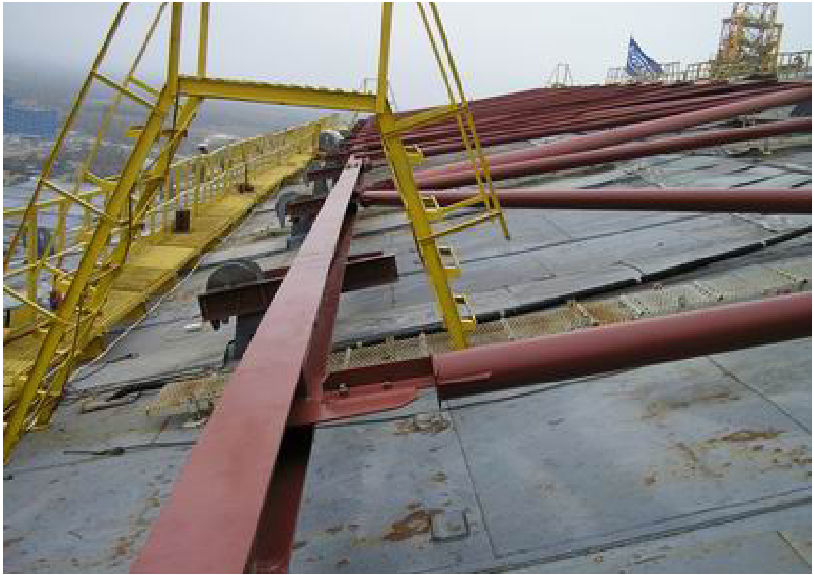
Fig. 5.18. Stabilisation of the south roofing zone.
