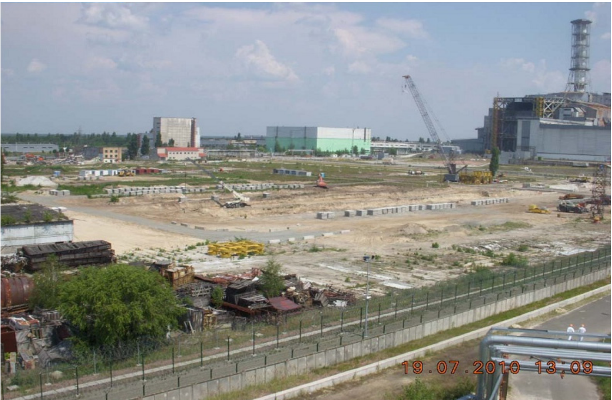
Fig. 5.21. NSC Construction Site Preparation.
