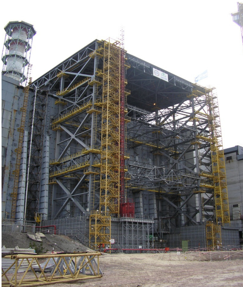
Fig. 5.17. SO western zone stabilisation.
