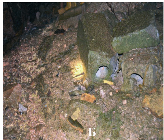
Fig. 5.11. Spraying of dust suppression solution (A) and protective polymer coating (B) of fragments in the SO inner space.
