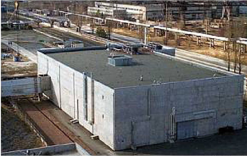
Fig. 5.29. Liquid Radwaste Treatment Plant.
