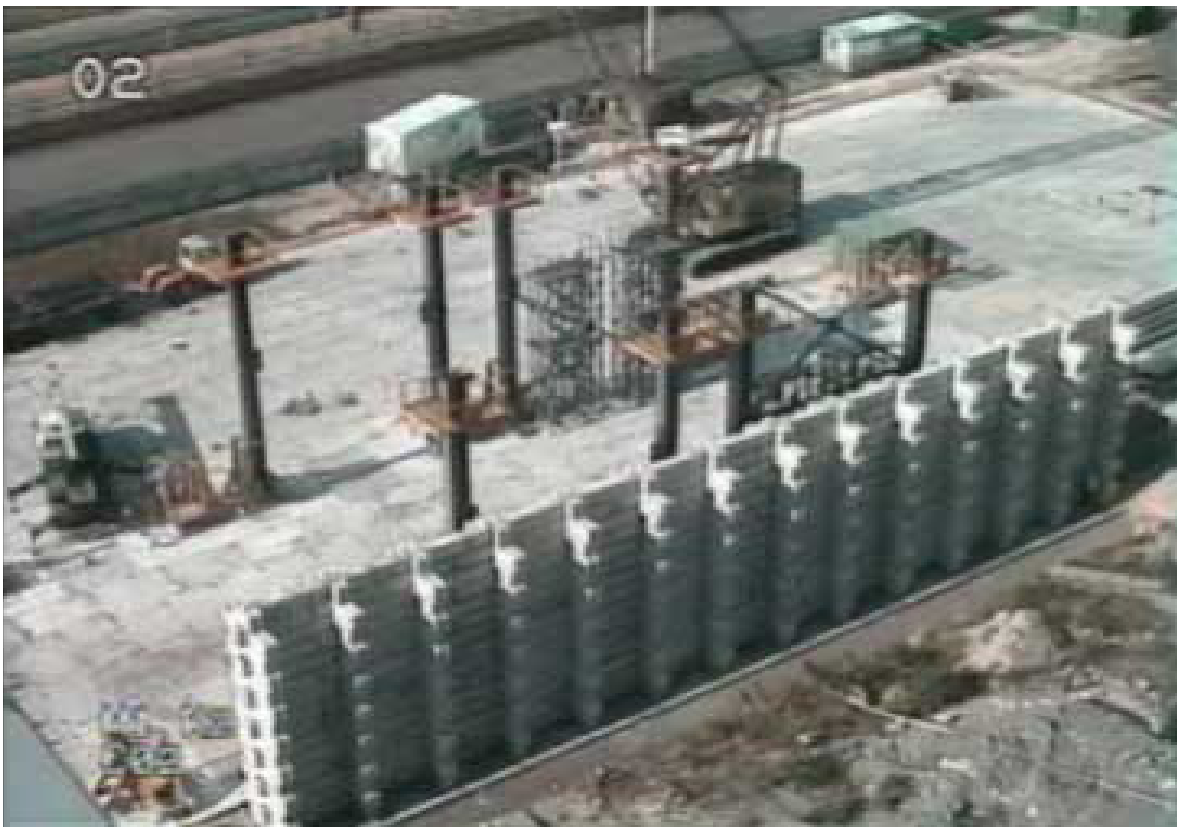
Fig. 5.19. The protective concrete wall.
