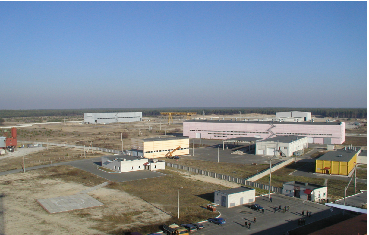
Fig.6.1. General view of the 'Vektor' Complex Commissioning Stage One.
