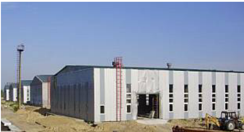
Fig. 5.31. Complex for producing metal drums and reinforced concrete containers to store radioactive waste.
