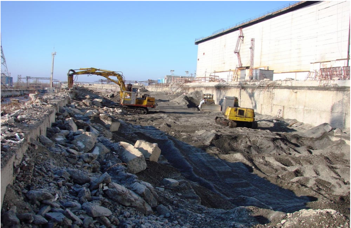
Fig. 5.20. Pioneer Wall Berm removal.
